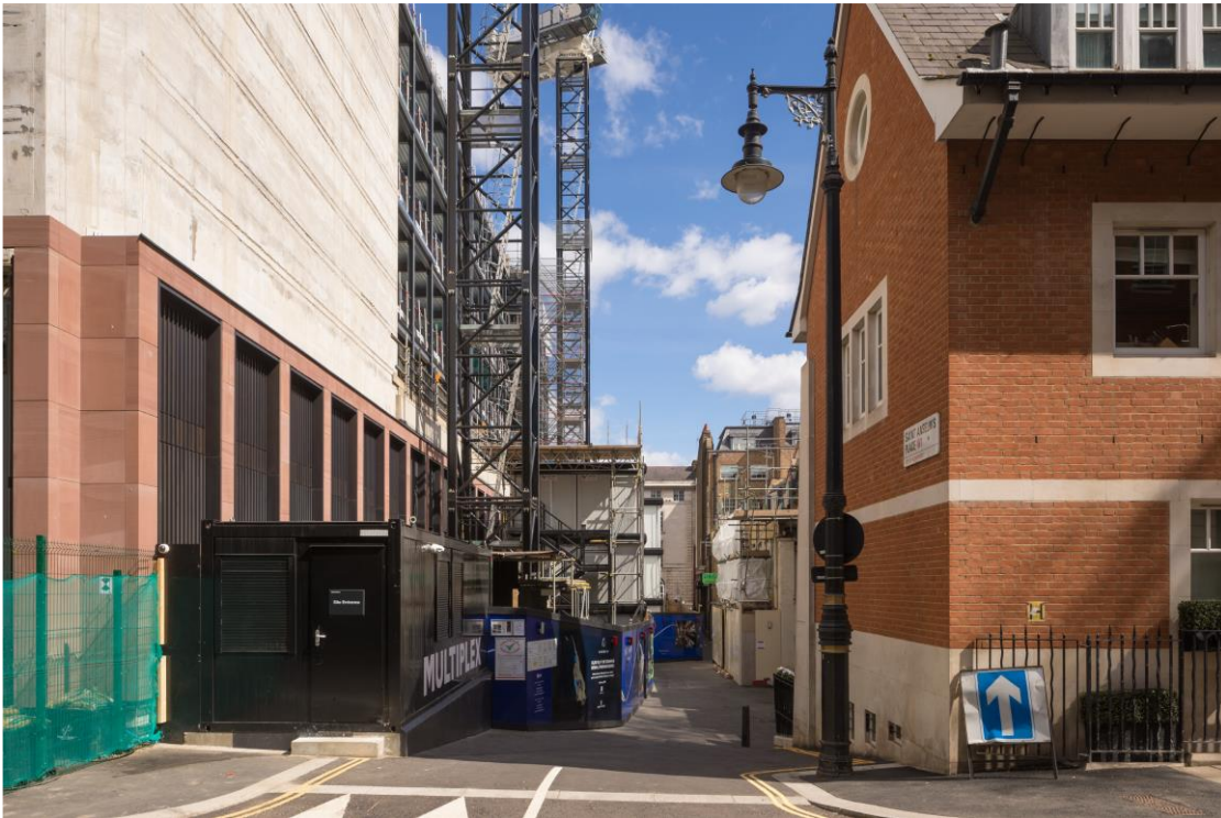
Existing view looking east from St. Anselm's Place
