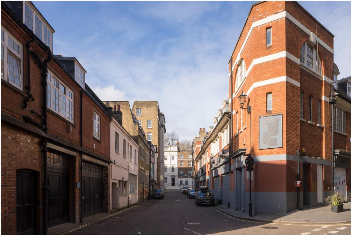
Existing view from South Molton Lane looking west along Davies Mews.
